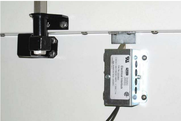
ELECTRO - MECHANICAL DOOR LOCK
