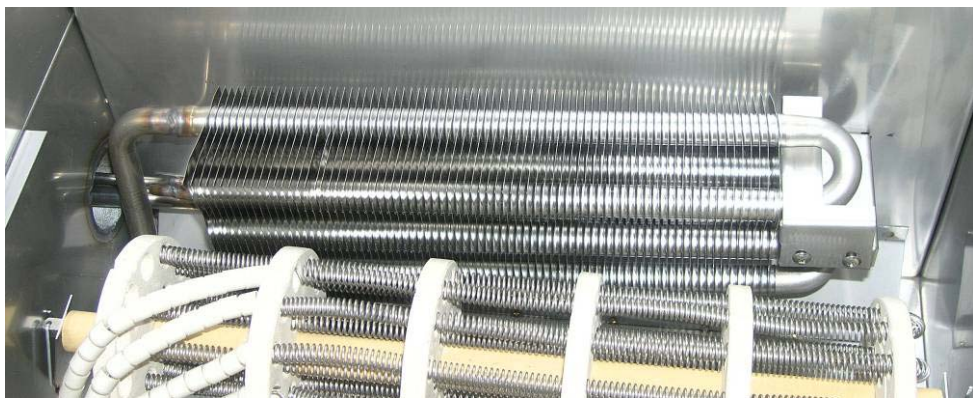
WATER-COOLED COOLING COIL
