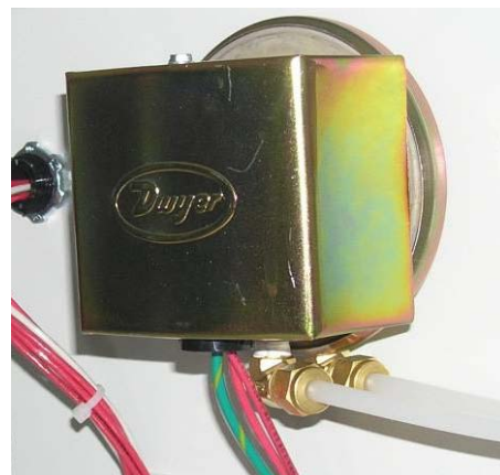
DIFFERENTIAL AIR PRESSURE SWITCH
