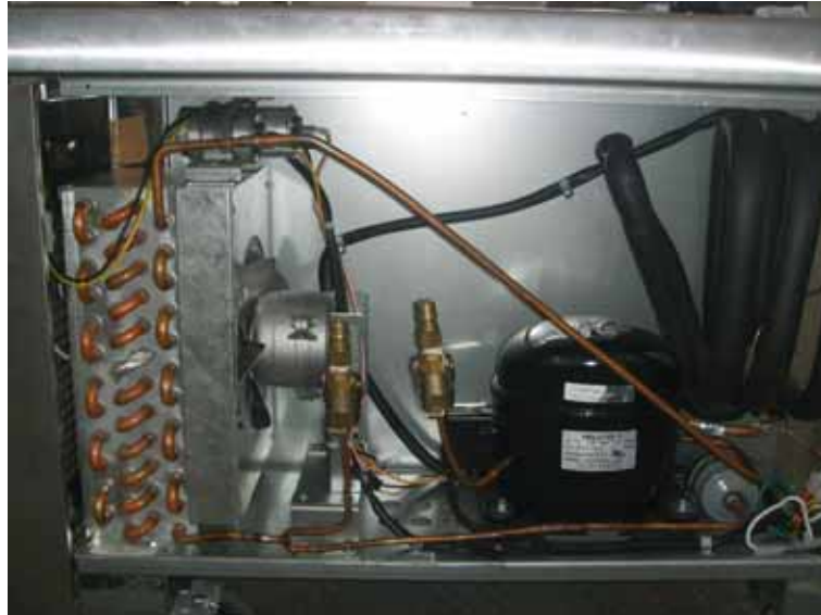
CONDENSING UNIT ASSEMBLY TCBE-52SDR
