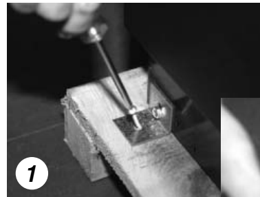
1 Removing bracket from skid.
