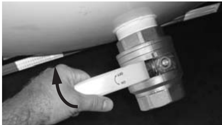
Figure 5-21. Close the tank drain valve.
