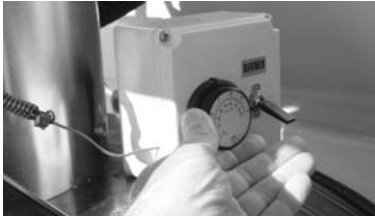
Figure 5-65. Set the water heater thermostat.
