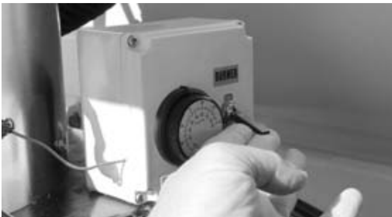
Figure 5-64. Push the power switch up to turn on the water heater.
