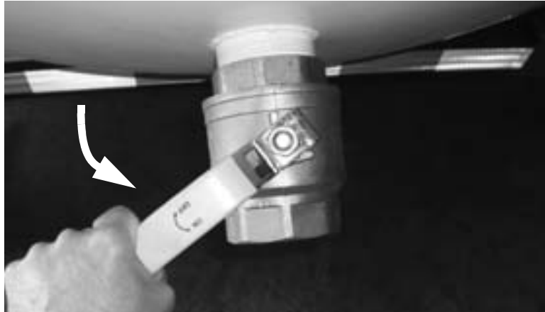
Figure 5-19. Open the tank drain valve.
