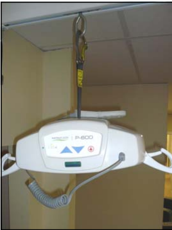
Figure 8A - Photo showing connection of lift hook directly to the eyelet of the trolley.
