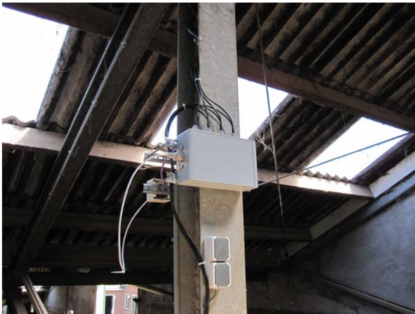
Fig. 18: Base station mounted to pillar
