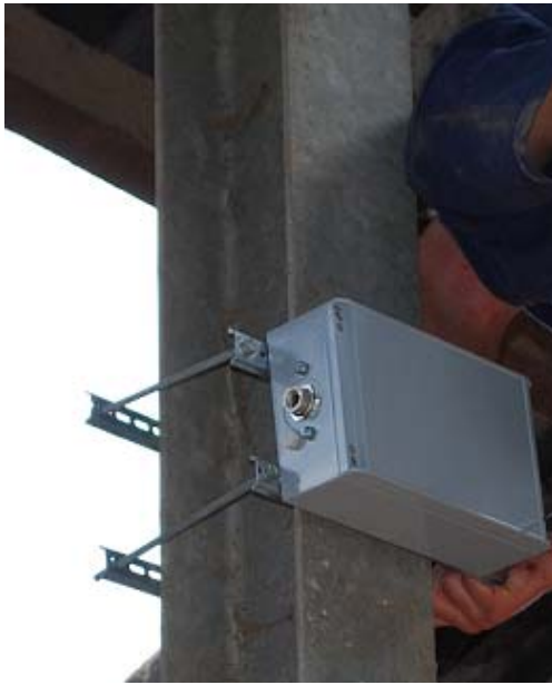
Fig. 19: Fixation using perforated metal plate
