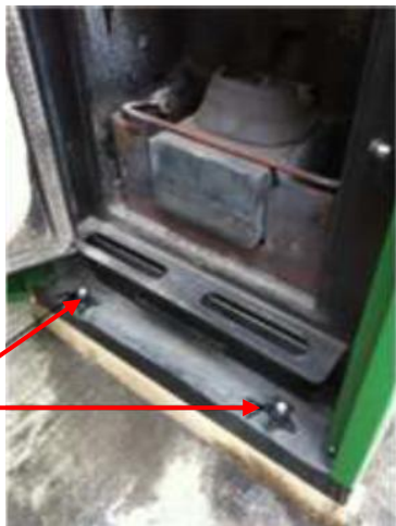
Unscrew locking nuts
