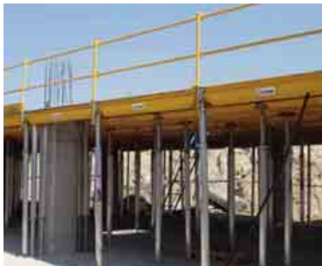
▲ Detail of Handrail post assembly
