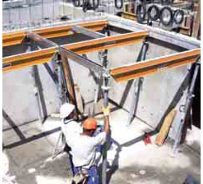
▲ Grid assembly for CC-4 Ply System
