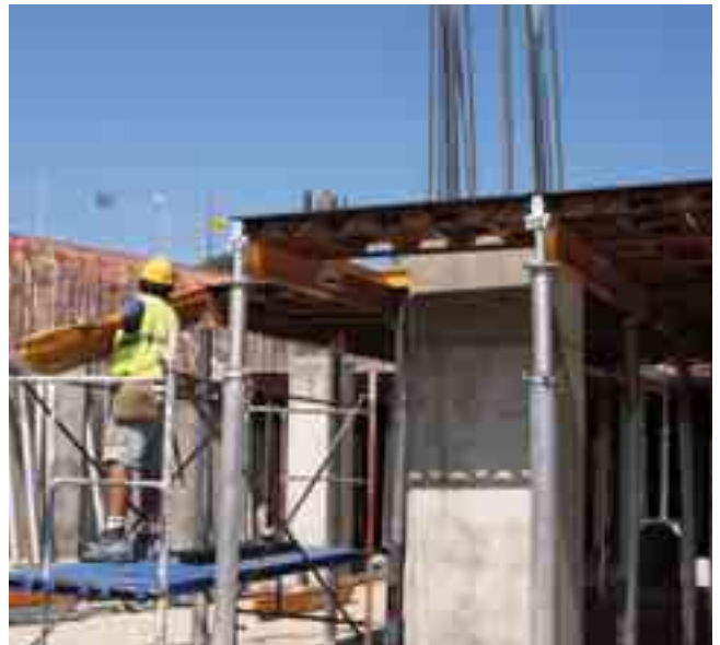
▲ Beams CC assembly
