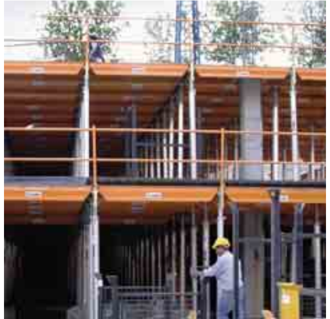
▲ Perimeter railing to provide safety during the execution process ▲
