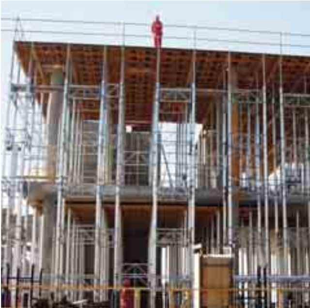
▲ Perimeter railing to provide safety during the execution process ▲
