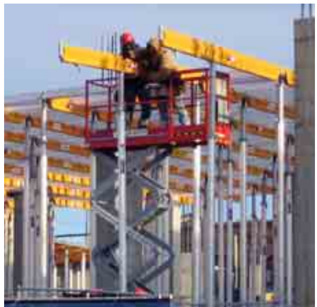
▲ Perimeter beam CC assembly
