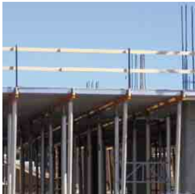
▲ Perimeter beam CC, which incorporates a tube for the Safety handrail on its end ▲
