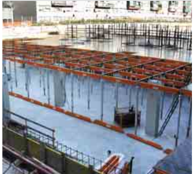
▲ Assemble the grid
