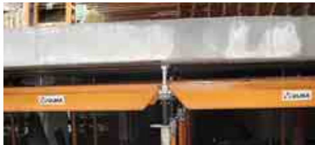
▲ CC-4 Panel System in dismantling phase
