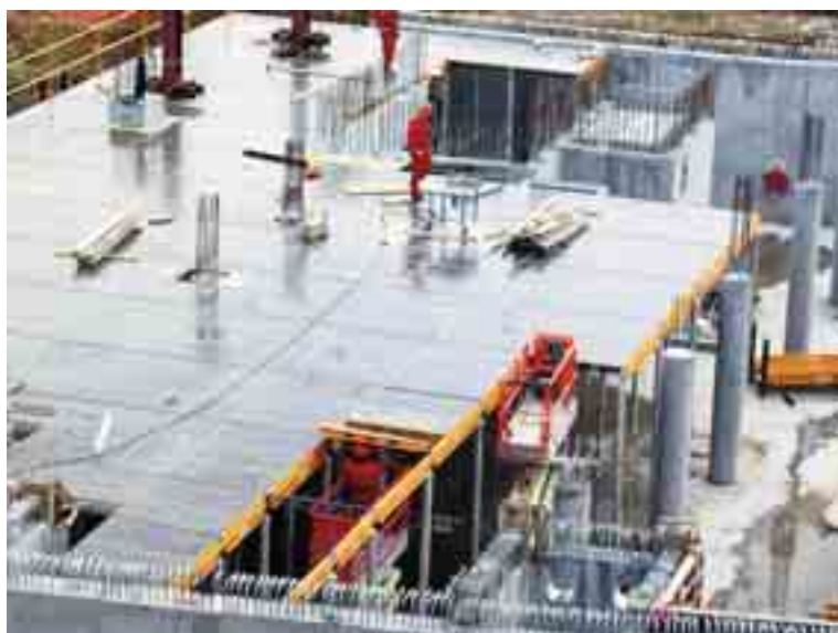
Mounting the Panels CC from ▶ lifting platforms
