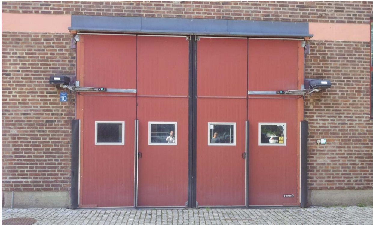
Figure 25: Metal garage door used for the distance measurements
