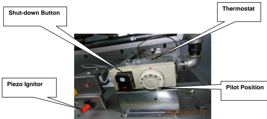
3. While pressing the ignition button down, use a lit match or piezo ignitor to ignite the pilot. Continue to press the knob down for about 30 seconds. If the pilot does not stay lit when the ignition button is released, repeat the lighting procedure and keep the ignition button down longer. Adjustment of pilot flame may be necessary.
