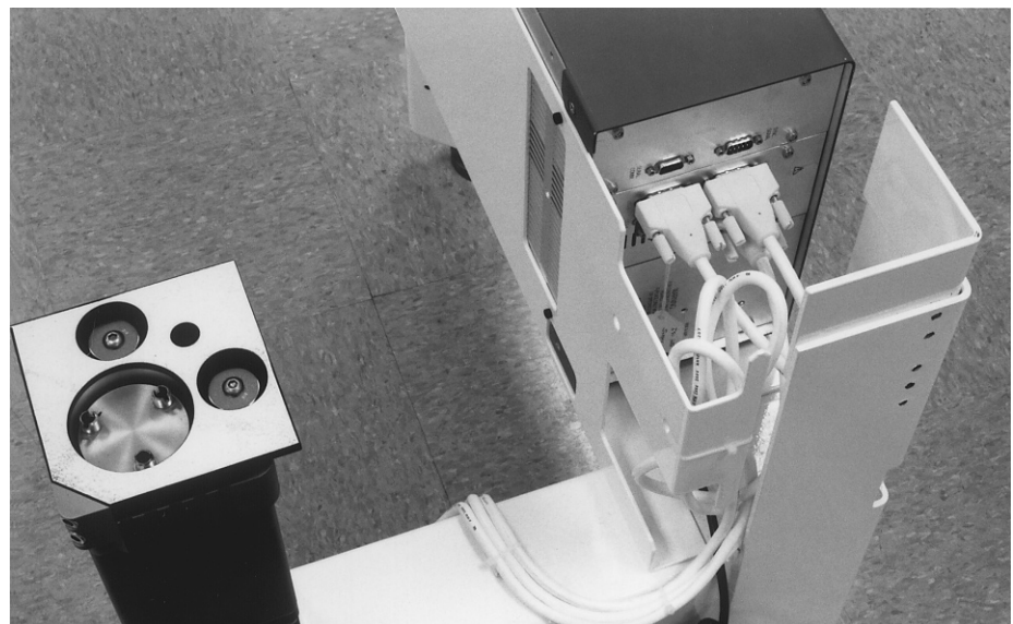
Figure 2.5 — Installing the Controller and Cabling
