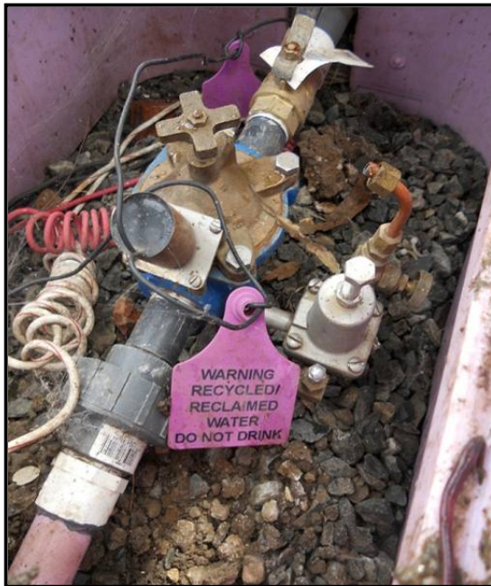
Tagged remote control valve
