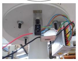
Once the ceiling plate has been fitted, it will be necessary to ensure that it is balanced on the vertical plane. This can be achieved by adjusting the  $2^{nd}$  level of nuts (the adjusting nut). Once this adjustment has been done tighten the  $1^{st}$  level of nuts down to the ceiling plate to lock the plate into position.
