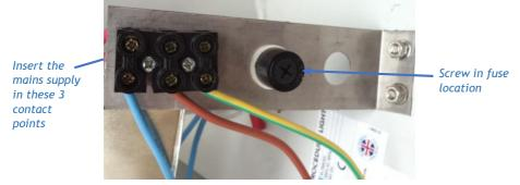
The mains supply lead will need to be wired into the central terminal block as shown above.
