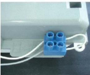
**Low Voltage Room Thermostat:** This picture shows the terminal block, which is located at the bottom left hand side of the control panel cover, to which the room thermostat must be fitted.
