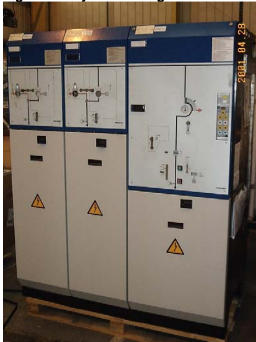
Figure 6: Physical arrangement of an RMU arrangement
