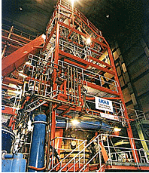
FIGURE 2.1.1. The blast furnace body.
