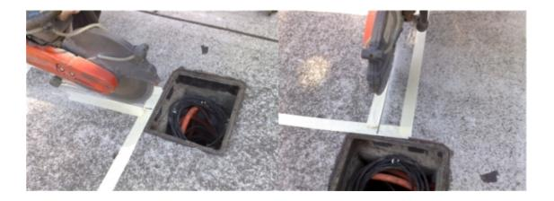
5. Clean loop area using broom or air-blower. When using an adhesive to secure pad, area MUST be free of dust and moisture.
