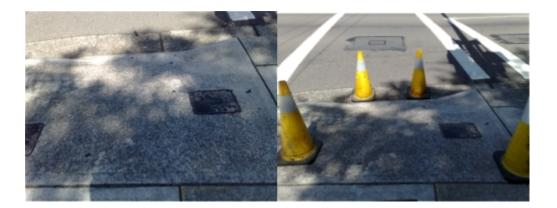
2. Lay loop pad onto pavement and mark-out using masking tape or similar. This will help to keep the surrounding pavement clean of adhesive.
