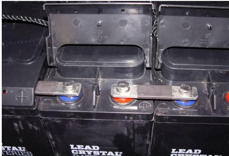
**Figure 13-1: Battery Terminals Connected with the Terminal Linking Bar**
