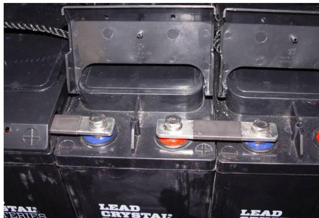
Figure 9-10: Battery Terminals Connected with the Terminal Linking Bar
