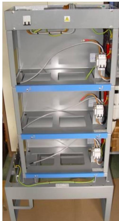
**Figure 3-2: Battery Expansion Cabinet Modules (Cabinet removed)**
