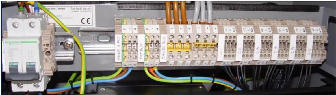
**Figure 9-9: UPS Connection Panel**
