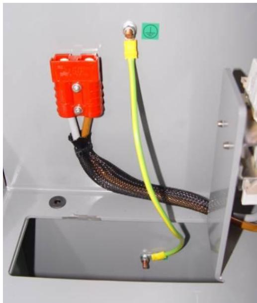
**Figure 9-6: Earth Connection between Battery Housing modules**
