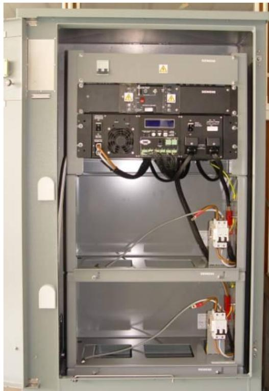
**Figure 9-7: UPS Housing mounted on Battery Housing within Cabinet**
