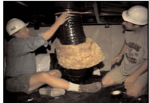
Fastening the inner lining of the crossover duct to the collar
