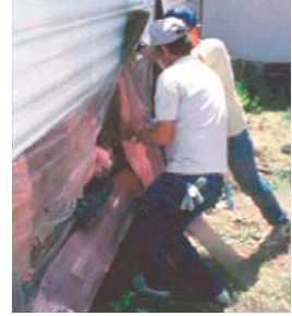
Stuffing fiberglass batts into a sidewall
