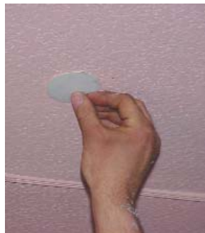
Plugging the ceiling hole
