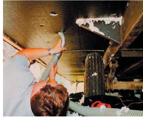
Blowing insulation into the floor cavity
