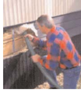
Blowing wall insulation
