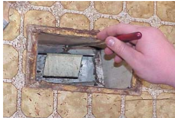
Inspecting the duct with a hand-held mirror
