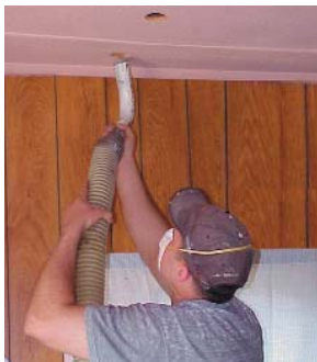
Blowing insulation through the ceiling
