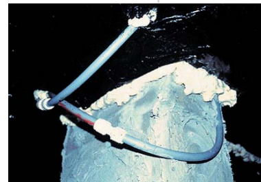
Bottom board penetrations sealed with patch and foam
