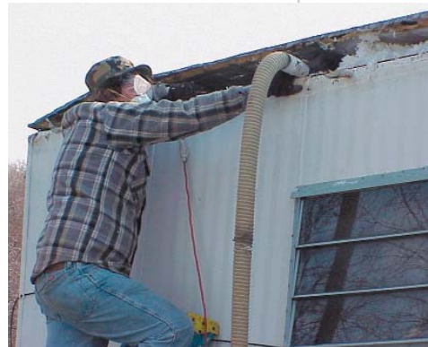
Blowing insulation into the roof
