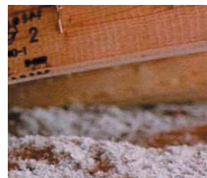
Loose fill insulation
