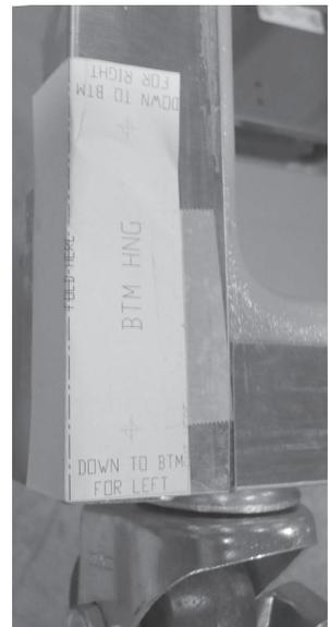
Bottom hinge template down to unit bottom
