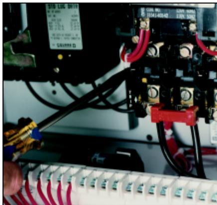
Figure 57: Tripping the Overload Relay
