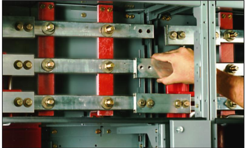
Figure 19: Aligning the Splice and Bus Holes
