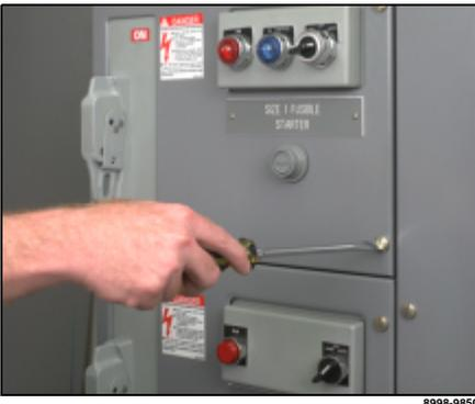
Figure 39: Loosening Captive Quarter-turn Fasteners
