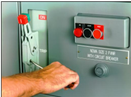
**Figure 60: Operating Door Interlock Defeat Mechanism**
