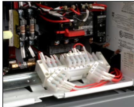
Figure 69: Power Leads Connected to Power Terminals
