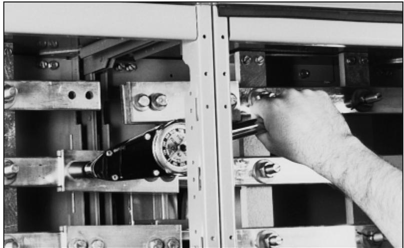
Figure 20: Torquing the Bolts
