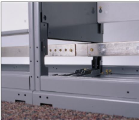
Figure 27: Ground Bar Bolt Replaced
