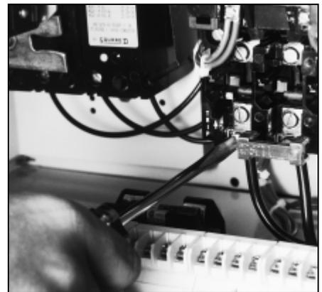
Figure 58: Tightening Electrical Connections
