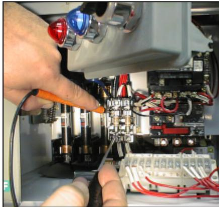
Figure 54: Inspecting Fuses
