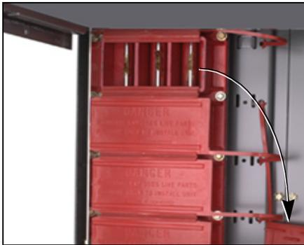
Figure 65: Removing the Manual Bus Shutter
