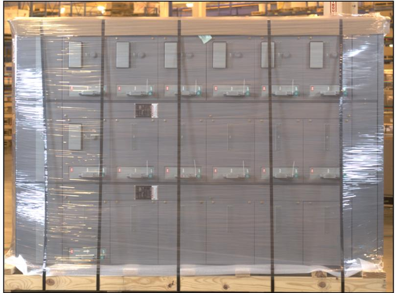
**Figure 1: Packaged Motor Control Center**
