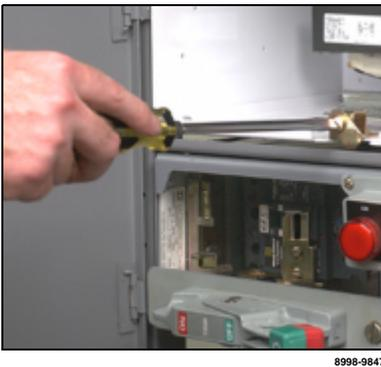
Figure 40: Releasing the Lock-in Device (when supplied)
