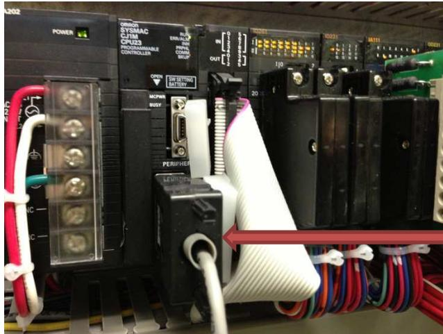
Disconnect the LCD cable from main processor CJ1M.
