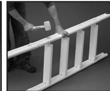
**#3:** Place a rail assembly on top of treads so the rail openings align with the tread ends and tap rail down.
