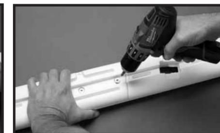
**#2:** Connect the Upper and Lower Outside Rails together using two #20 x 1/4" x 7/8" bolts and two 1/4" hex nuts. Repeat to assemble second Outside Rail.
