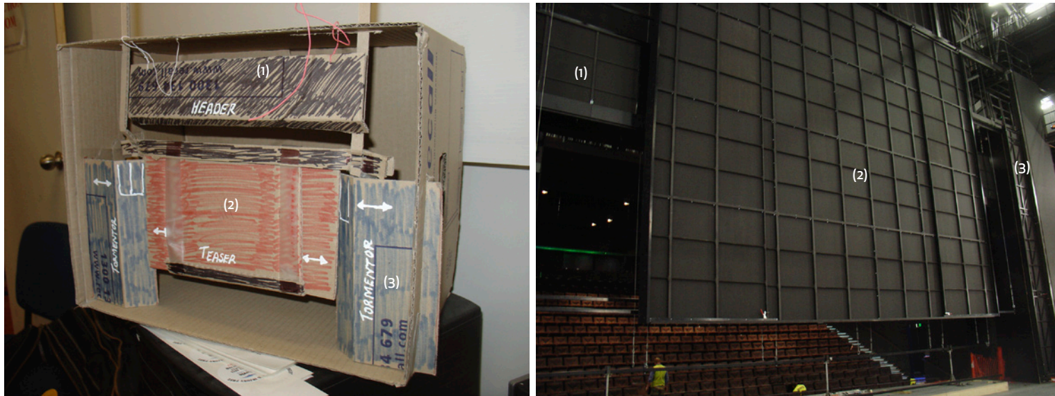
Left: Not only was stage terminology and technology initially unfamiliar to the team from project builder Bovis Lend Lease, but the concept of the re-sizeable proscenium opening (that could move in so many directions at once) was hard to pick up from the engineering drawings. To make the concepts abundantly clear, the builders knocked up this down 'n' dirty, not-even-slightly-to-scale, model. Right: A view from the stage showing what the cardboard model was actually describing: (1) The proscenium header; (2) The teaser; (3) The tormentor with its panels and Juliet balcony.
