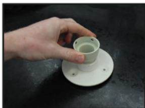
2. Using the bracket as a stencil, mark out the drill holes needed in the wall.
