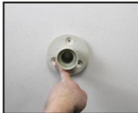
3. If feeding wires through the ceiling you will need to drill a hole through the ceiling for the wires to go. However, if placing through the bracket, you can just feed through the side.
