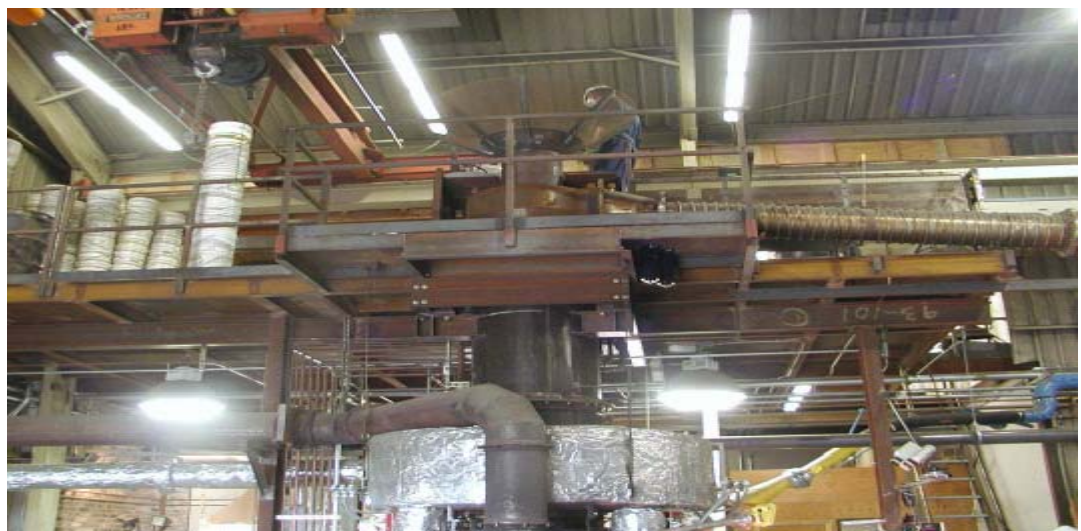
Figure 5-30: Charging Deck of the Cupola at ALRC
