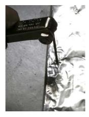
**Fig. 11, 12:** Find the set screws under the foil insulation and push through with an allen wrench.
