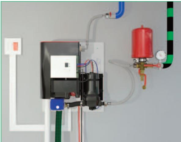
Connect the single length of the suction hose to the control panel unit, as shown, using the fittings provided. It is essential that this is water tight as any leaks will allow air into the system, resulting in pump failure and from this other potential problems can occur.
