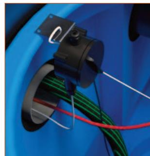
In cases where the cables are not long enough to reach the panel, run the cable into a waterproof junction box which needs to be mounted on the bracket in the turret as shown. Within the junction box connect it to a length of the specified cable and run that through the duct to the panel.
