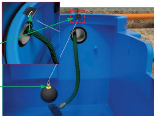
Attach the provided steel rope to the L shaped bracket and through the loop on the top of the float.
