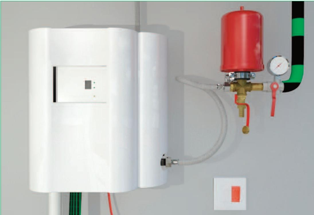
The StormSaver control panel is the central hub of the system. All the rainwater must pass through here on its way to the points of use. The control panel is the place where all the different pipes and hoses connect up, and should be considered when choosing its location within the building. The unit comprises of the pump, a small water storage tank, a pressure vessel and the electrical control panel which enables the whole system to function and includes the display panel.
