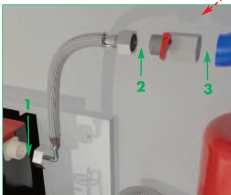
1. Connect stainless still braided hose to the mains water inlet valve on the unit.(supplied)
