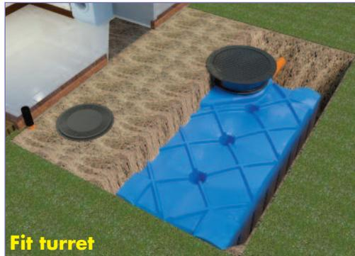
Top soil, clay, loam and other types of cohesive soils and materials with sharp edges are not suitable filling materials. Carefully backfill type 1 aggregate to all sides and up to at least 100mm above the top of the tank, compacting at every 100mm interval. It is also important to compact the material down into the column supports in the tank.
