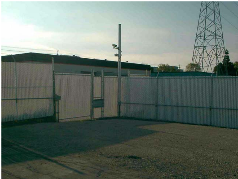
Figure 14: Example PIR Barrier
