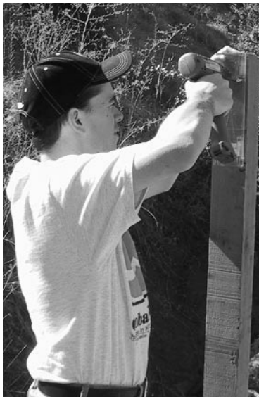
Screw the mounting bracket onto the post, making sure the bracket is level.
