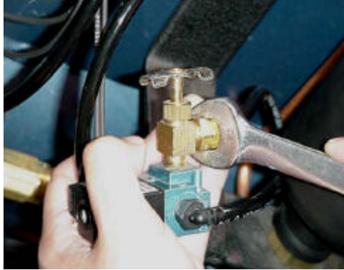
Unscrew nut counter-clockwise
