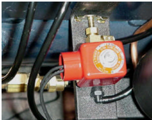
position housing on valve
