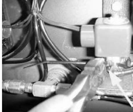
zip tie all wires and hoses
