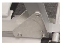
(4) Now raise the other ends in the vertical position so that the snaplock pin at the elbow joint snaps in place.
