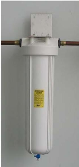
When the water is being drawn from a lake or other surface water source, the MAYTAG Whole Home Water Filtration System is equipped with an External Sediment Filter. Not all Systems include this device.
