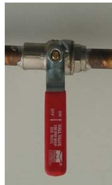
Photo 2b: Ball valve: closed position
