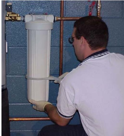
Photo 6. Disassembling the External Prefilter Housing
