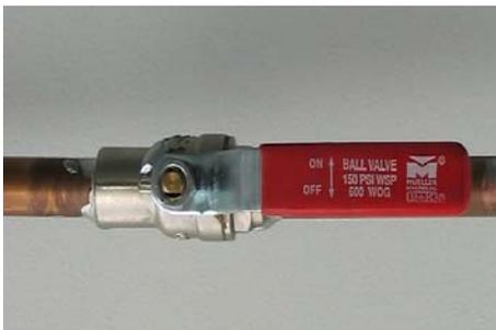
Photo 2a. Ball valve: open position
