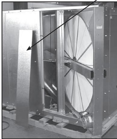
This panel must be removed before the energy wheel can slide out. (ERV-522 only)
