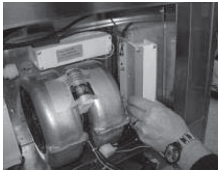
3. Position capacitor box as shown.
