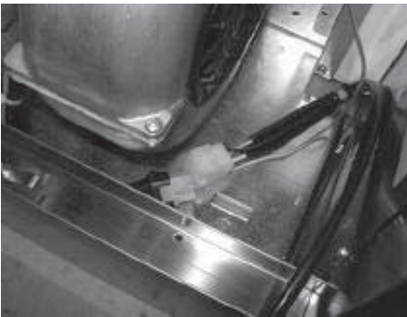
7. Attach short capacitor connector to blower connector.
