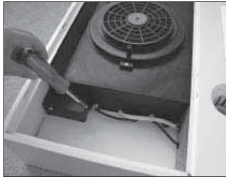
2. Remove cover from junction box to gain access to the electrical wiring.
