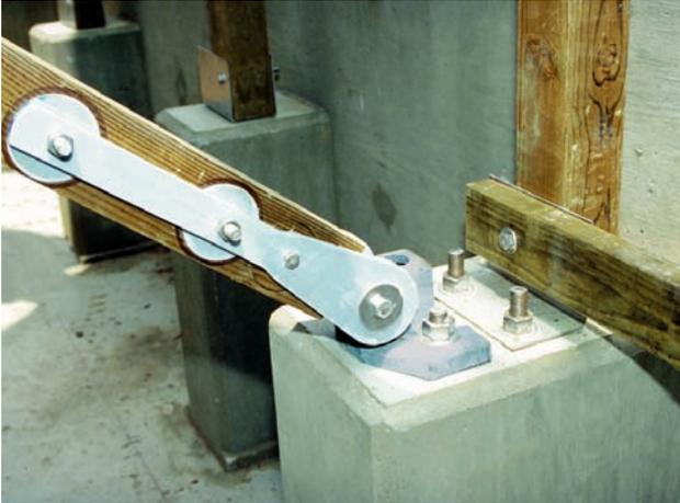
All structural framing connections use 1/2" dia. galvanized machine bolts with either fiber-reinforced nylon shear connectors or FRP connector straps.
