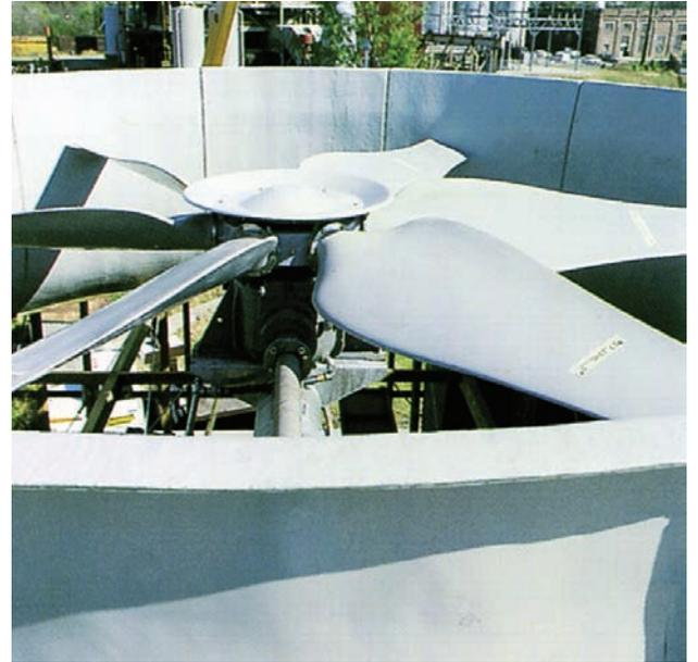
Fans operate inside structural GRP (glass-reinforced polyester) eased-inlet fan cylinders designed and applied to maximize fan performance. Cylinder height varies from 3'-5" to 7'-0", depending on fan diameter. Cylinders less than 6'-0" tall include galvanized welded fan guards. (See Access and Safety on page 7.)
