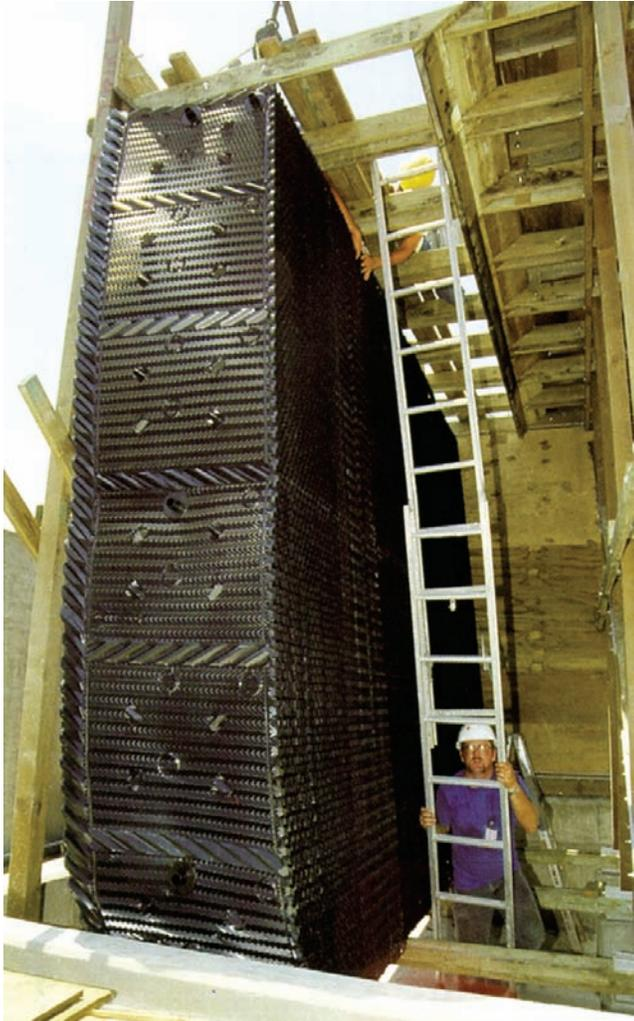
Fill sheets are vacuum formed 15 mil (.015") thick polyvinyl-chloride (PVC) capable of service at hot water temperatures up to 125°F. Stainless steel structural tubes resting in stainless steel hangers support the fill, and PVC tubes control alignment. Series 1000 fill includes two stainless supports, and Series 1200 fill uses four stainless supports. This system also holds the bottom of the fill sheets above the cold water basin floor to simplify basin cleaning.
