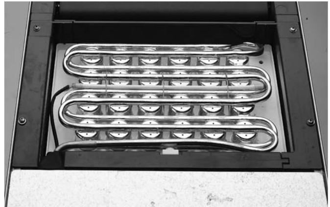
**Pour Scale Remover Over The Evaporator Section**
