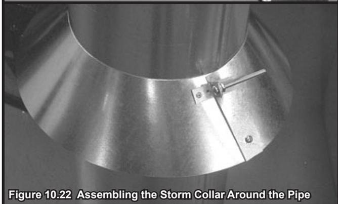
Figure 10.22 Assembling the Storm Collar Around the Pipe
