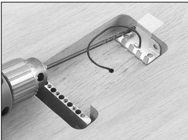
**Figure 24.** Drilling the spring hanger mounting holes.
