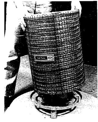
Fig. 27 — Removing Outdoor Coil
