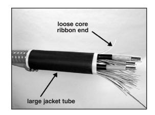
3.2 Slide a 3M<sup>™</sup> cold shrink splice body onto each core of **Cable X** with the loose core ribbon end going on the cable first, away from cable end.
