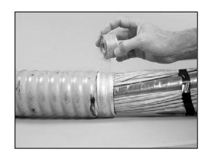
5.2 Wrap an end of the ground continuity braid around exposed armor and applied 24 tape on one cable end.
