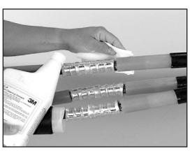
4.5 Apply red compund on cable insulation, making certain to fill in edges of cable semi-cons.
