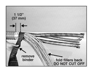
2.3 Cut the phase cores to the appropriate length.
