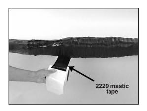
6.6 Cover the applied 2229 mastic with two half lapped layers of 88 tape.
