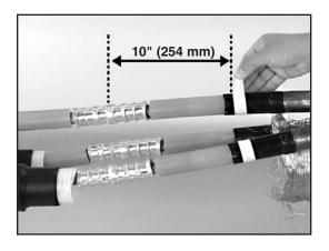
4.3 Position cold shrink copper connector adapter **over CENTER of connector.** Shrink the adapter near center of connector by pulling and unwinding the loose core ribbon end in a counter-clockwise direction.
