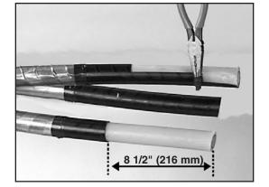
Remove cable insulation from conductors ends of both Cable X and Cable Y.
