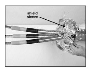
3.4 For 1/0 through 3/0 AWG connectors, or connectors with an O.D. between 0.51–0.76" (13,0–19,3 mm): Slide the cold shrink adapter tube with the WHITE CORE onto the insulation with the loose core ribbon end going on first, away from the cable end.
