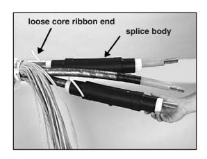
3.3 Expand metallic shield sleeves and slide one onto each core of **Cable Y**. Compress the ends of each shield sleeve together next to the cable armor or jacket, away from the prepared conductor ends.
