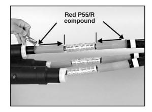
4.6 Position each splice body over the connector and align the leading end of the rubber part with the center of the marker tape.
