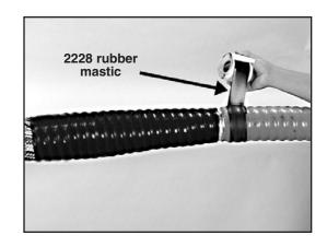
6.3 Install a Cold Shrink jacket tube on each cable with the leading end just covering the 2228 mastic and the tube extending toward the splice bodies.
