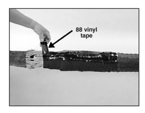
6.5 Apply two half-lapped layers of 4" wide 2229 tape over applied vinyl tape in splice center. Overlap ends of Cold Shrink jacket tubes 2" (51 mm).
