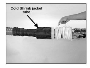
6.4 Apply one half lapped layer of 88 tape over the unjacketed area in splice center. Do not overlap the Cold Shrink jacket tubes.
