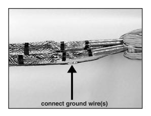
4.10 Unfold the cable fillers and reestablish their lay between the cable phase cores. Hold the fillers in place with a band of 33+ vinyl tape.
