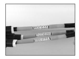
4.2 Apply a tape marker to core semi-con insulation screens of Cable Y (cable side which does not contain splice body) at a distance of 10"
