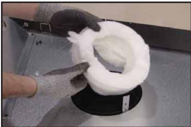
**Figure 7.6** Remove the insulation from the outer vent pipe. For rear venting there is no insulation in the outer vent pipe.
