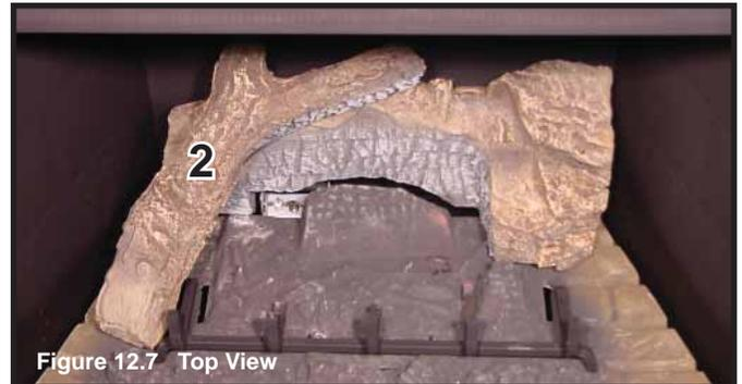
**STEP 4. Log #2 (SRV2103-108):** Place log #2 on top of the left side of log #1. The bottom of this log has a slot in it that goes over the tab molded into the top of log #1. The left end sits behind the simulated ember cluster on the burner top.
