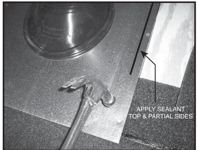
Figure 8.21 Slide Flashing Down, Secure & Apply Sealant
