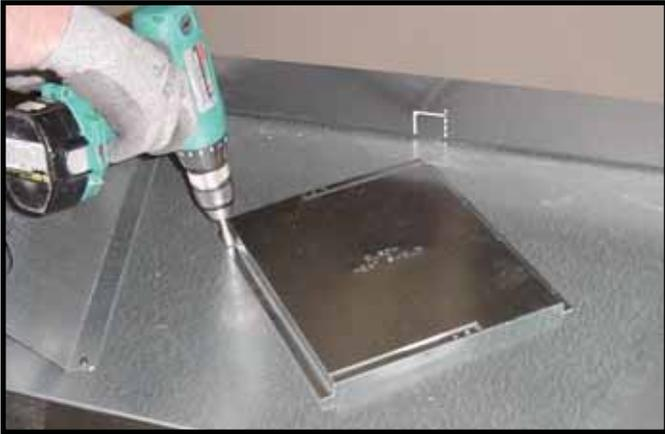
**Figure 7.1** For top vent, remove the two screws holding the elbow heat shield in place. Use this heat shield over the first elbow if applicable. For rear vent skip this step.
