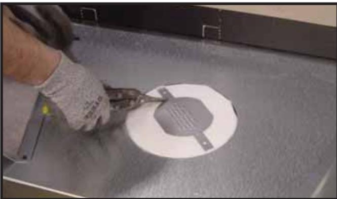
**Figure 7.2** Cut the seal cap strap across the rectangles next to the disk.
