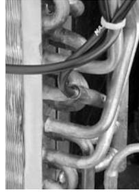
Prevents indoor coil from freezing and causing complaints due to lack of cooling. Frost can form on the indoor coil when the unit is operated in cooling when outdoor temperatures are low. The unit automatically shuts the compressor off until the indoor coil temperature warms to the point where frosting will no longer occur.
