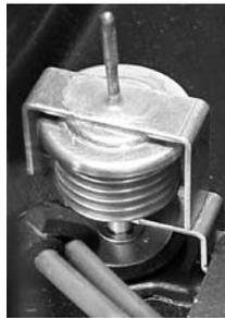
The most widely used method of disposing of heat pump condensate is with a "Temperature-Activated Drain Valve." This is a device mounted in the base pan of a heat pump unit with a bellows that expands on temperature rise and contracts with temperature drop. A shaft with a rubber plug on the end is connected to the bellows. When the outdoor temperature remains
