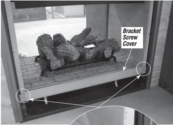
**Step 1 -** Remove the two #8 screws from the *bracket screw cover* on both sides.
