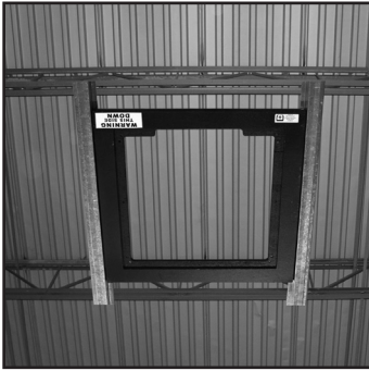
Fig. 4: Pre-installation ring on steel furring channel prior to drywall being placed.
