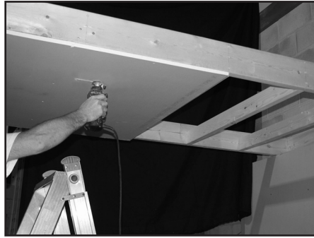
Fig. 5: Cutting drywall using the Rotozip™.
