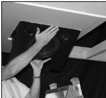
Fig. 7: Installing the subwoofer using the ledge to temporarily secure it.
