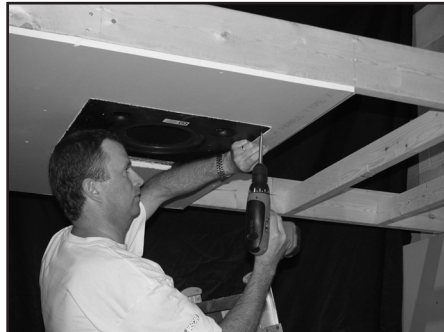
Fig. 8: Attaching the subwoofer to the pre-installation ring.
