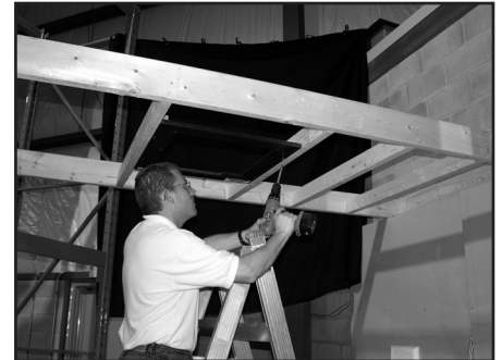
Fig. 3: Attaching pre-installation ring to blocking.
