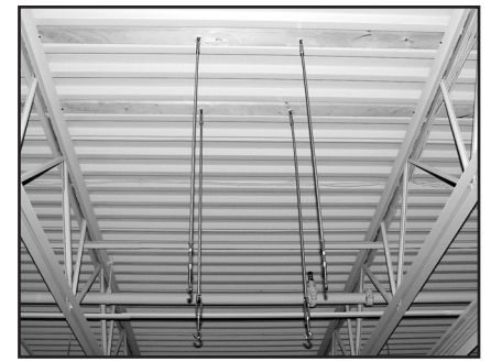
Fig. 13: Suspension points with turnbuckles installed.
