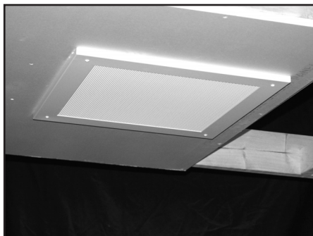
Fig. 10: Completed subwoofer installation.
