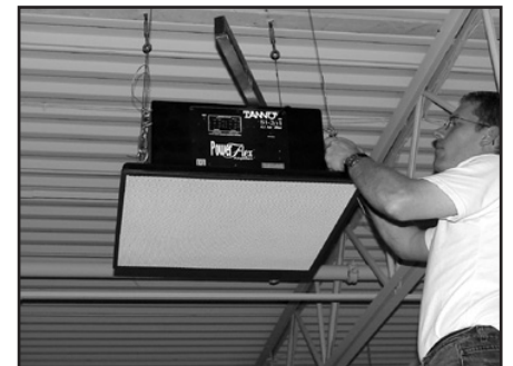
Fig. 16: Leveling the subwoofer.
