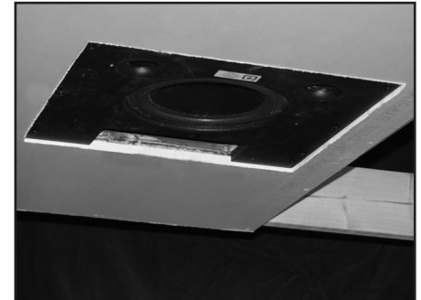
Fig. 9: Completed subwoofer detail.
