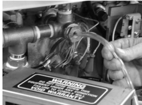
8. Feed the tubing through the access port in the boiler compartment.
