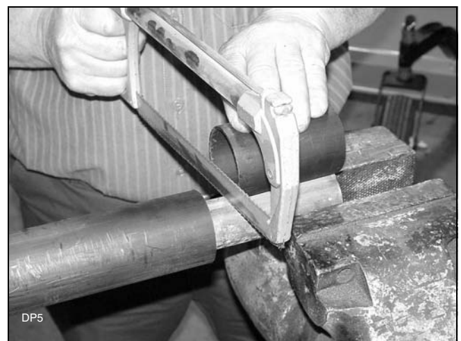
Figure 9. Cut Shaft to Length
