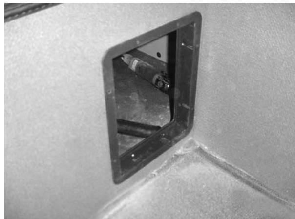
Figure 8 - Return air grill flange installed
