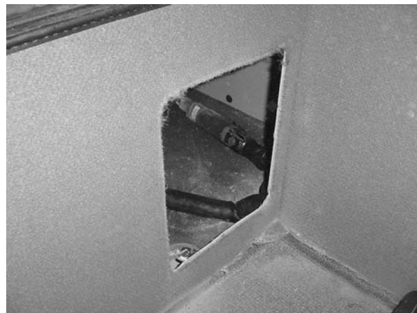
Figure 7 - Return air vent hole cut
