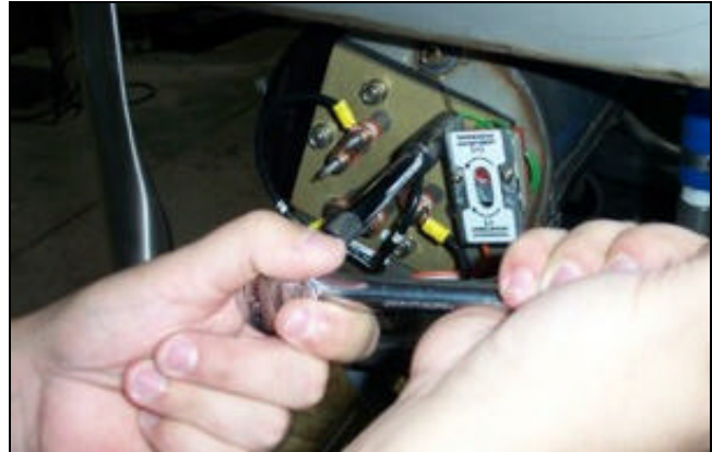
Removing the thermostat bracket/heater nuts.
