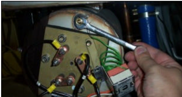
Removing the imperial brass fitting (Tempstar).
